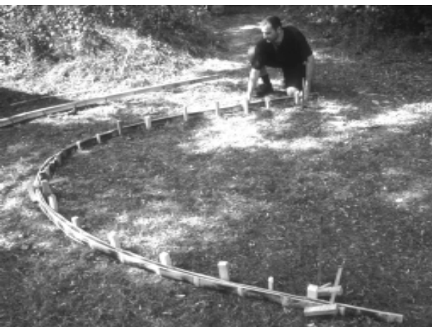
15-7 Construction of the arc with split bamboo
