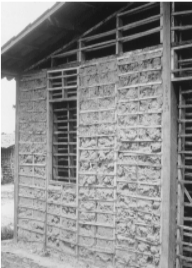
8-3 Prefabricated system CEPED, Brasil
