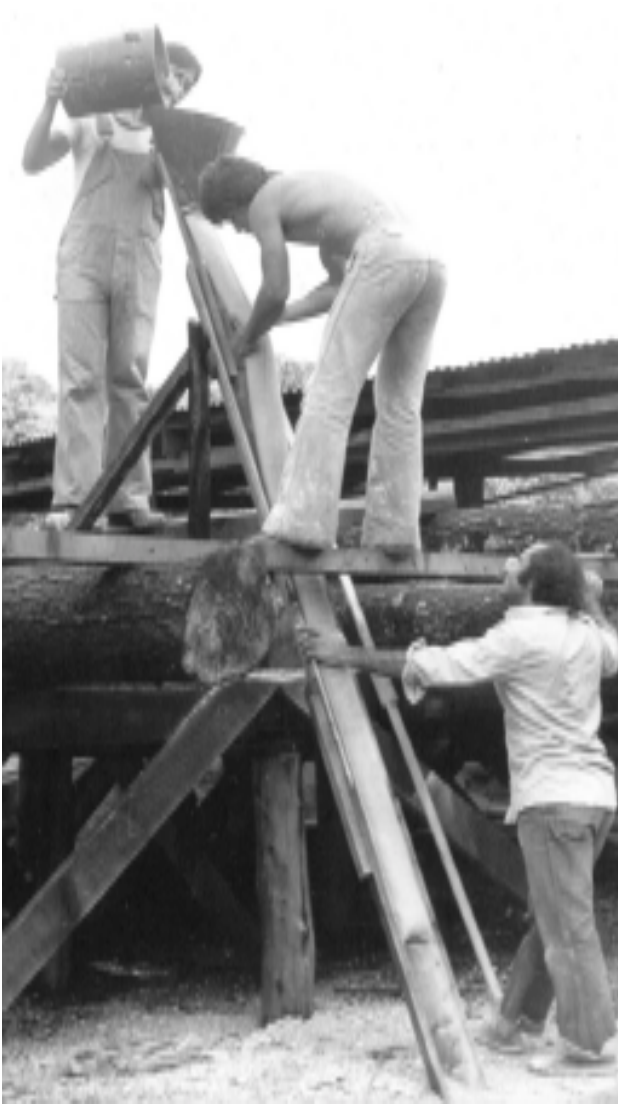
9-4 to 9-6 Filling and stacking of textile elements
