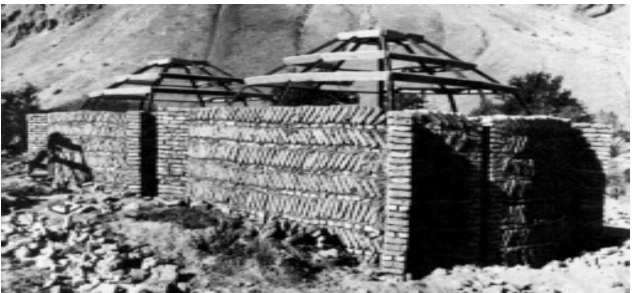
4-4 Earthquake-proof houses, Afghanistan (Sibtain 1982)
