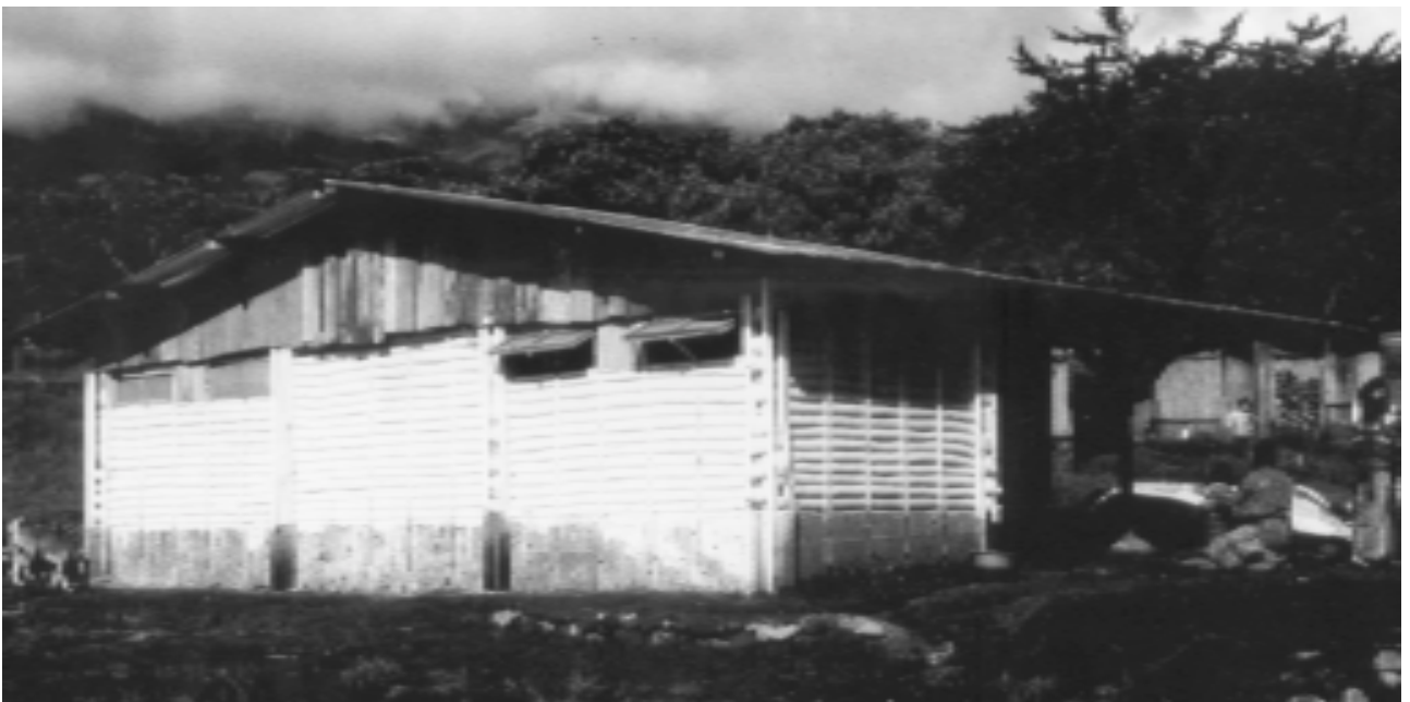
9-7 Earthquake resistant low-cost housing prototype, Guatemala 1978
