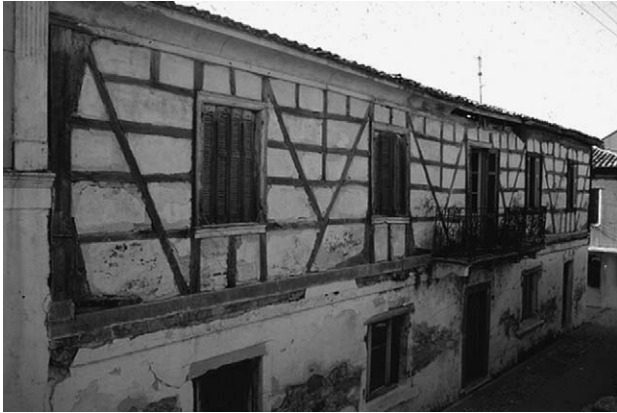
Fig. 7. Typical morphology of timber-framed walls.
