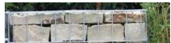
Photos from web of gabion basket retaining wall (above). The photo below shows how inconspicuous the wires can be if the basketing is of only a single layer of stone.
