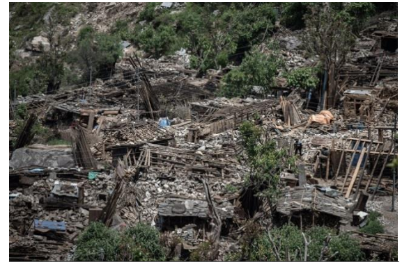
Destroyed rubble stone houses. (web)
